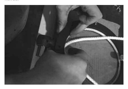
6: INSERT THE BOLT NEAREST THE HINGE AND TIGHTEN IT A COUPLE OF TURNS.
