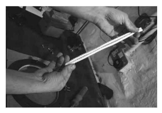
5: AND THEN PUSH THE CENTRE POINT OF THE ROPE IN BETWEEN THE DOOR FRONT AND THE GLASS IN LINE WITH THE BOLT NEAREST THE HINGE.
